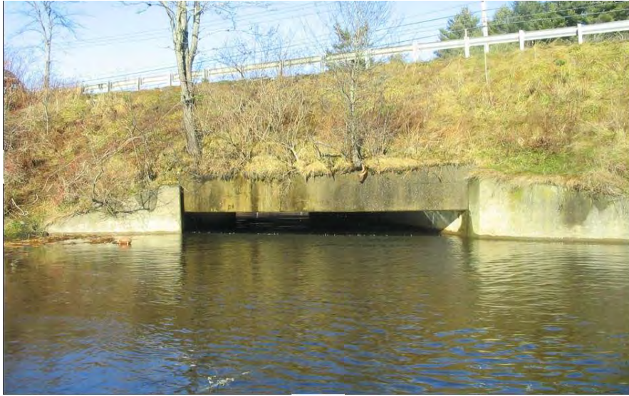
Figure 2. Bridge from downstream. MDOT inspection photo. Note low freeboard.
